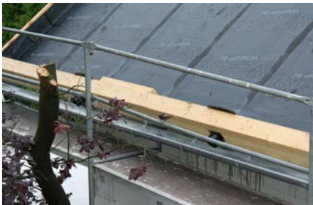
Wooden eaves up-stand before the waterproofing.
