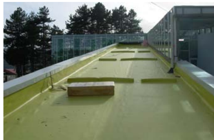
Waterproofed, interrupted shear barriers.
