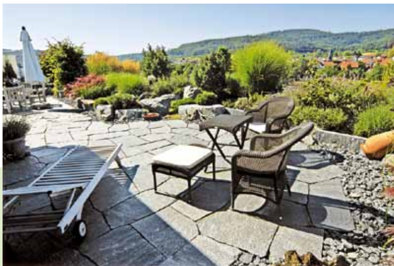
Intensive Green Roof
